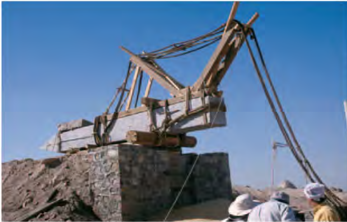
The raising derrick lashed to the obelisk waiting on the ramp.
