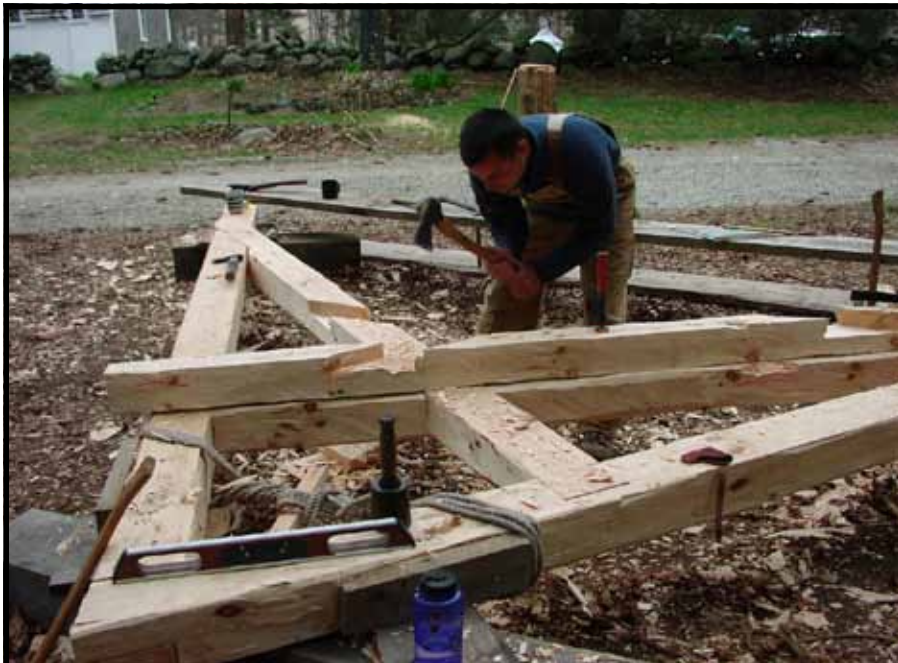
Gwozdziec timber frame roof workshop - Handhouse Studio - 2006
