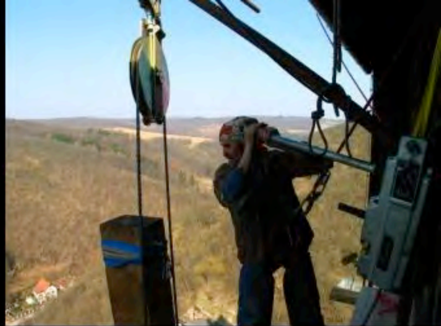
Lifting by hand with a come-along.
