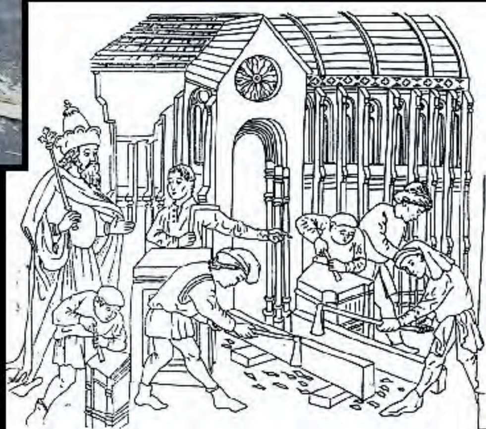
Hewing - long handled ax low position
