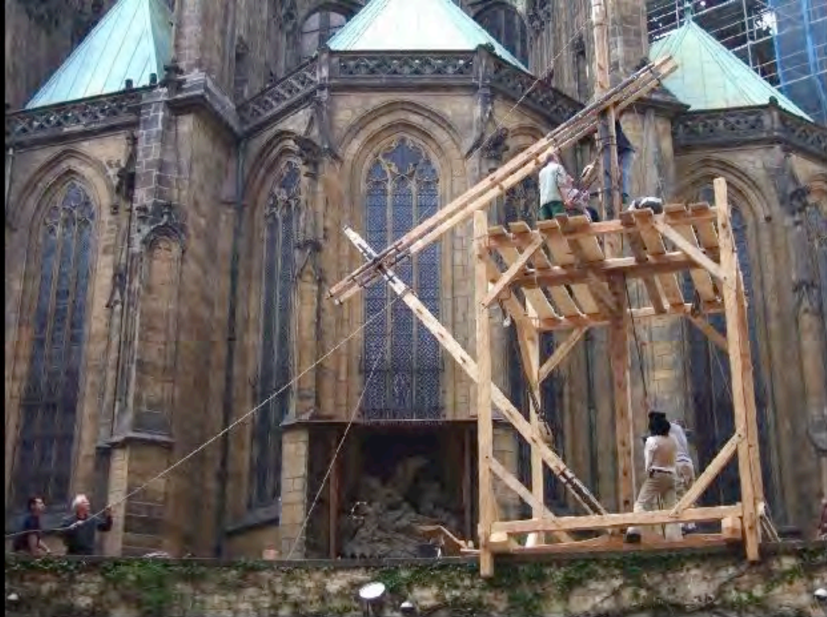
Raising and attaching the Lifting Arm to the Post
