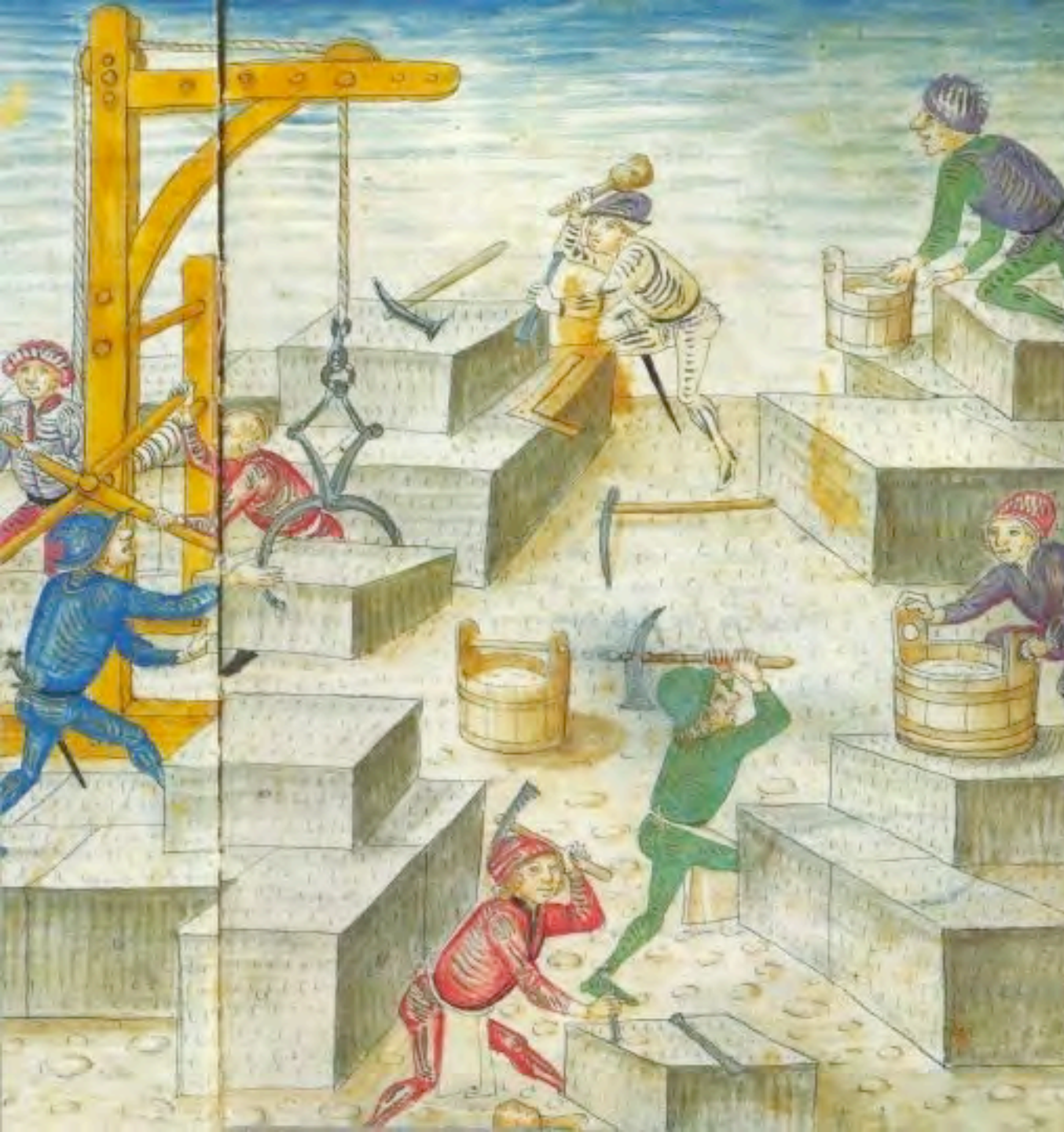
Lifting Arm with Windlass
