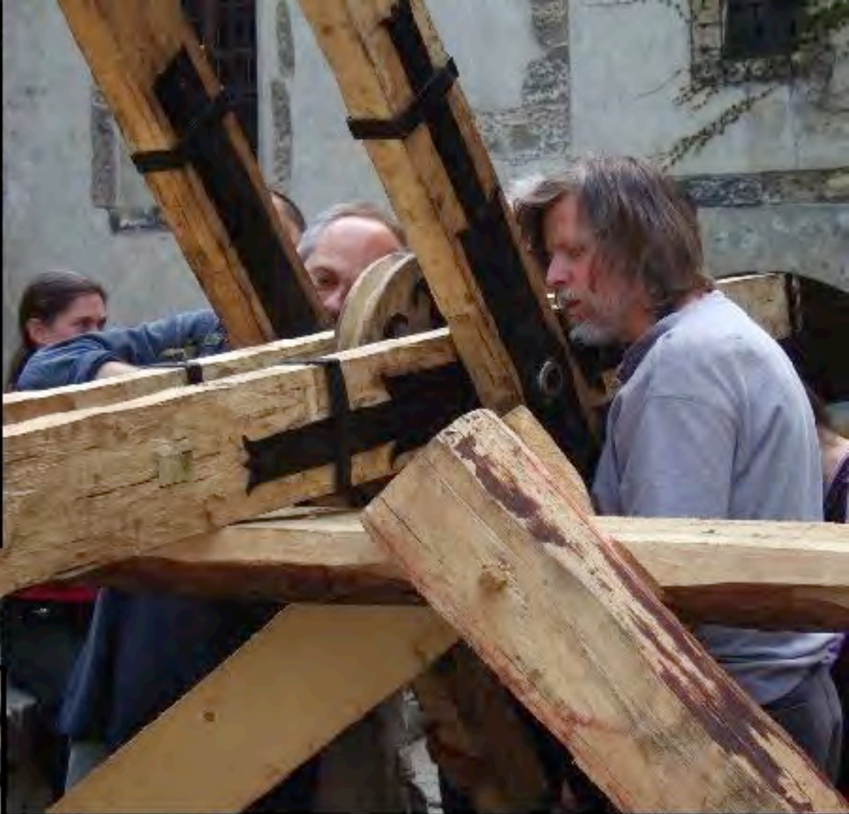
Setting the Sheeve in the Lifting Arm
