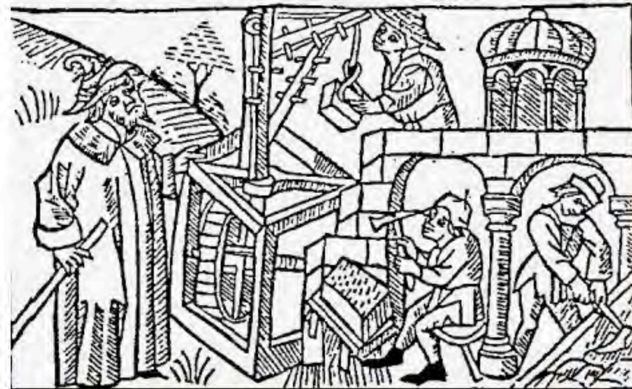
Example of Cage Crane - Strasbourg 1482.
