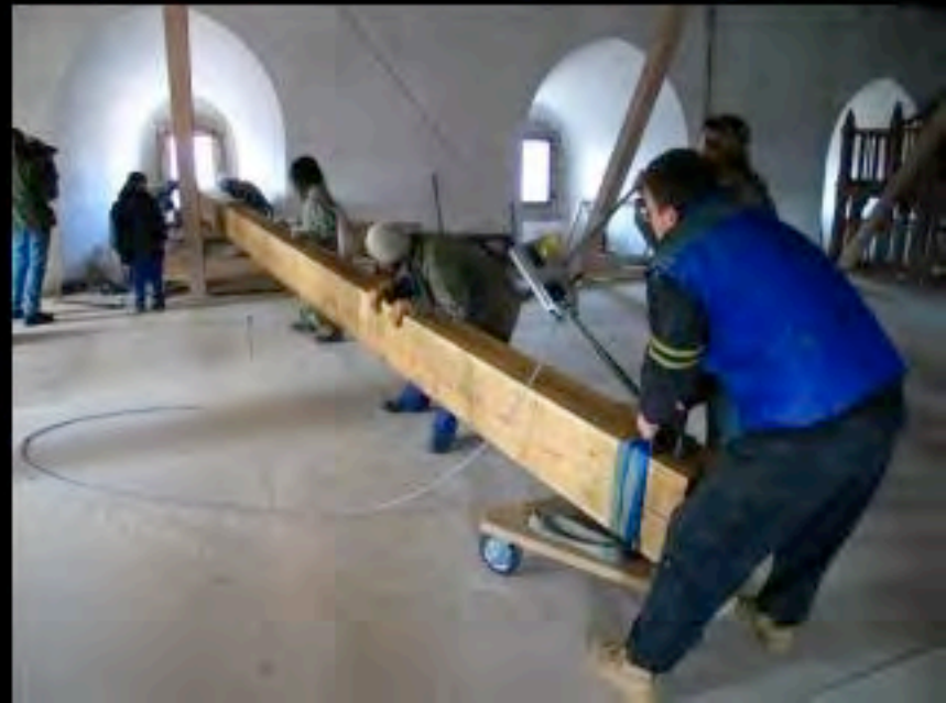
Lifting by hand with a come-along.
