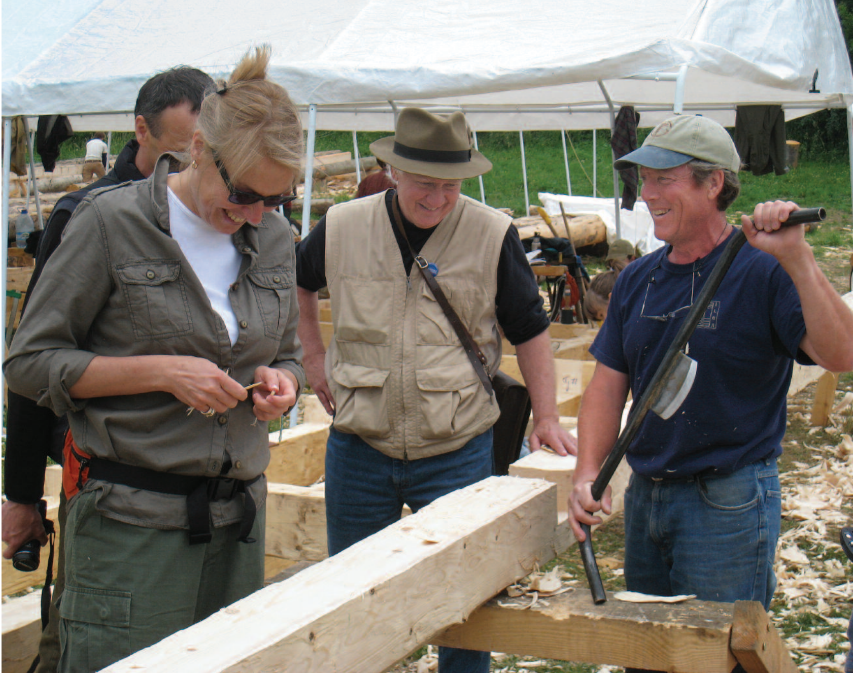
12 John Nininger, with drawknife, explains hollowing the underside of a squared log to fit neatly over the one below in a full-scribe hewn log wall. From left, Museum of the History of Polish Jews director Agnieszka Rudzińska and Gwozdziec project co-director Rick Brown.
