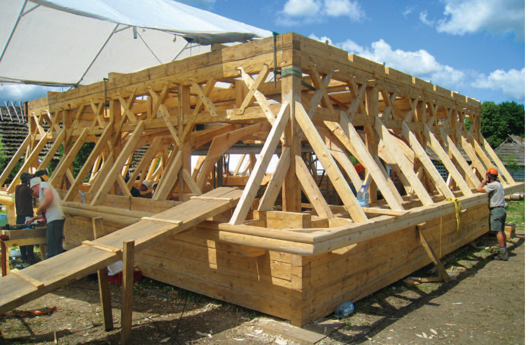
1 Short log wall and base of synagogue roof to be installed with remaining elements and finished interior in 2012 at Warsaw museum.
