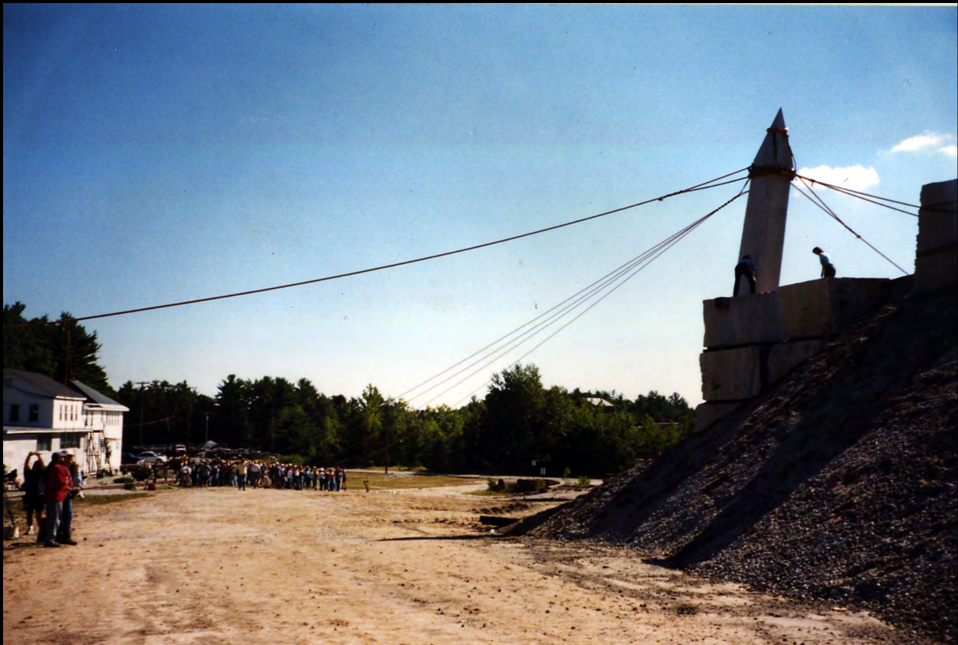
The final pull - Raising the obelisk from 75 to 90 degrees.
