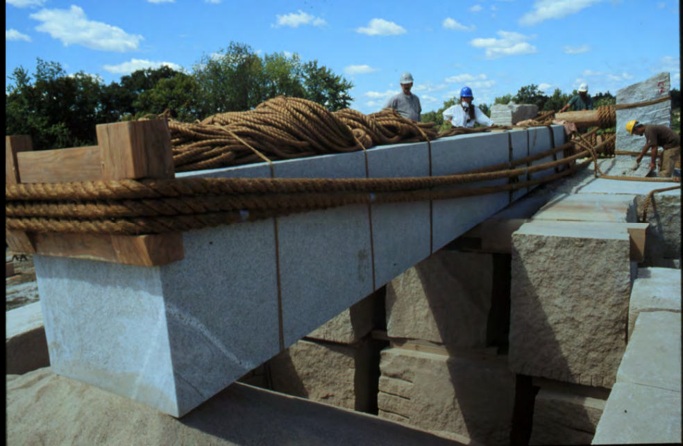
Guided rotation using 3" ropes and break blocks.
