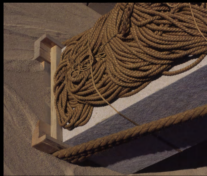
Fig. 3.21 Lowering ceiling blocks, suspended from three ropes, into the shaft of the Ka-tomb of Senwosret I at Lisht.
