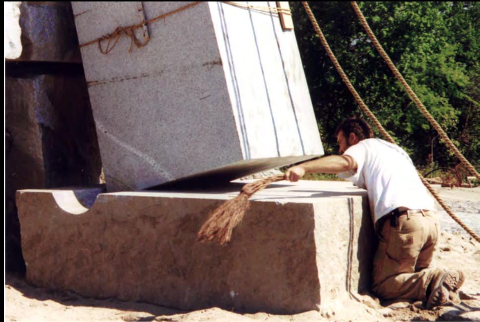
Cleaning sand from pedestal stone.
